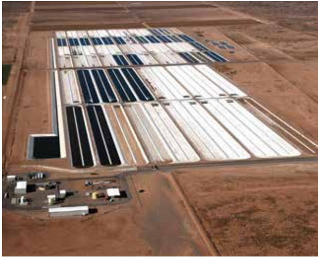
Algae facility in Columbus, NM
